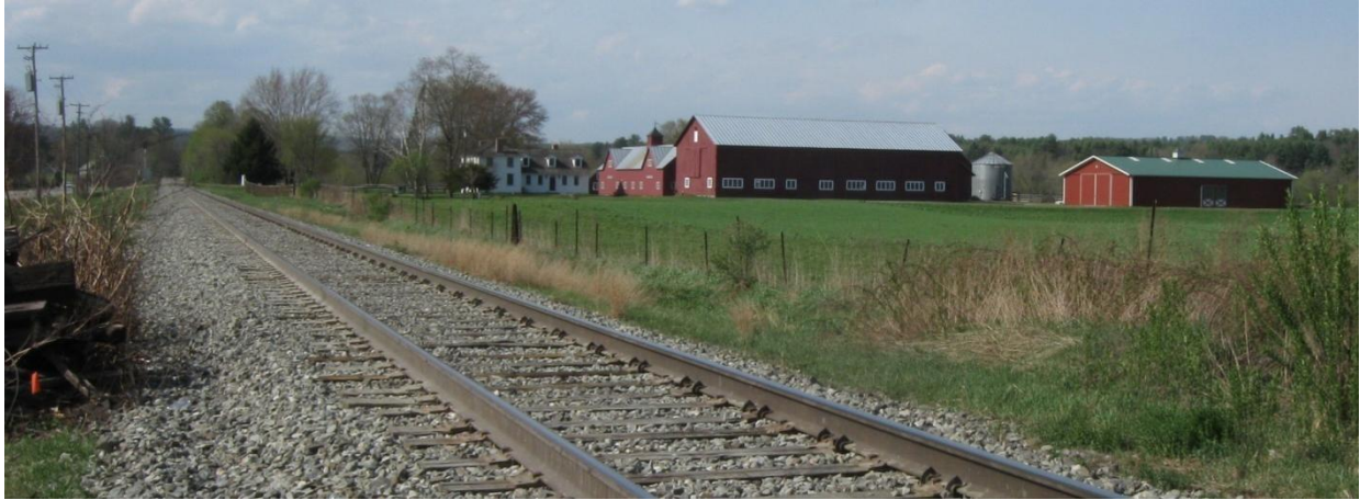
Rail in Windsor.
