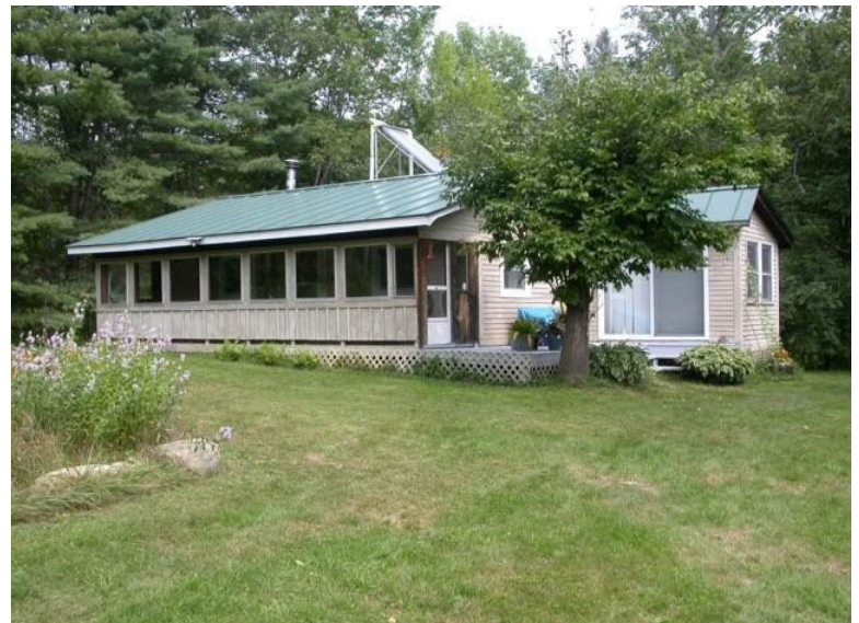
Figure 4: A solar hot water system (evacuated tubes) on a house in Weathersfield. (Julia Lloyd Wright)
