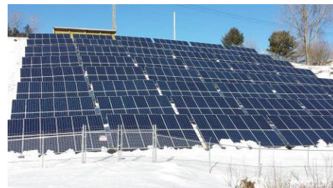
Figure 24: This is a photo of the Town-owned 150 kW solar project in Cavendish, an example of a perfectly sited project. Because it is not visible from any major public roads and has no neighbors, no landscaping is warranted. (Credit: Peter LaBelle)
