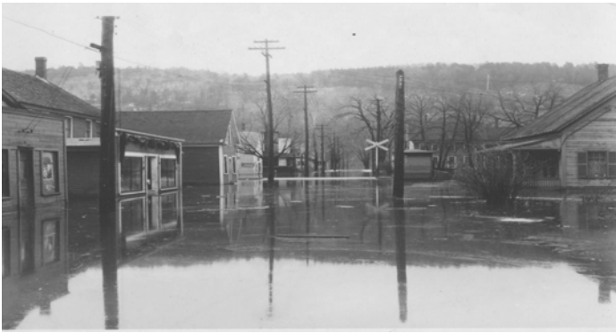
View of River Street from flood (1927)
