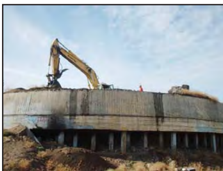
Construction underway at Kendall Yards.
