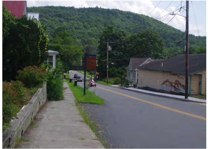
Use of both sides of the blades to confirm wayfinding towards the Windsor-Cornish Covered Bridge is recommended.
