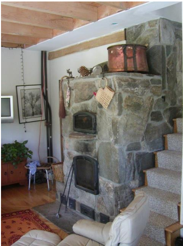
Figure 6: A masonry heater is a very efficient way to heat a home with wood. (Peter Hudkins)
