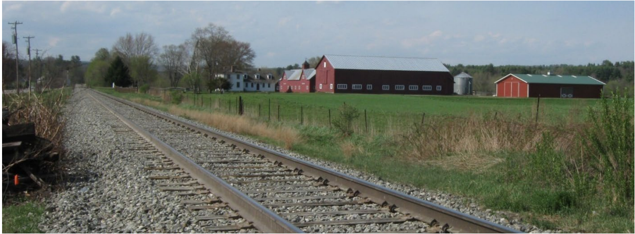
Rail in Windsor.
