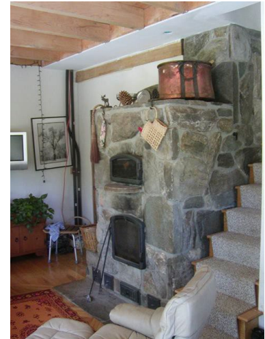
Figure 6: A masonry heater is a very efficient way to heat a home with wood. (Peter Hudkins)
