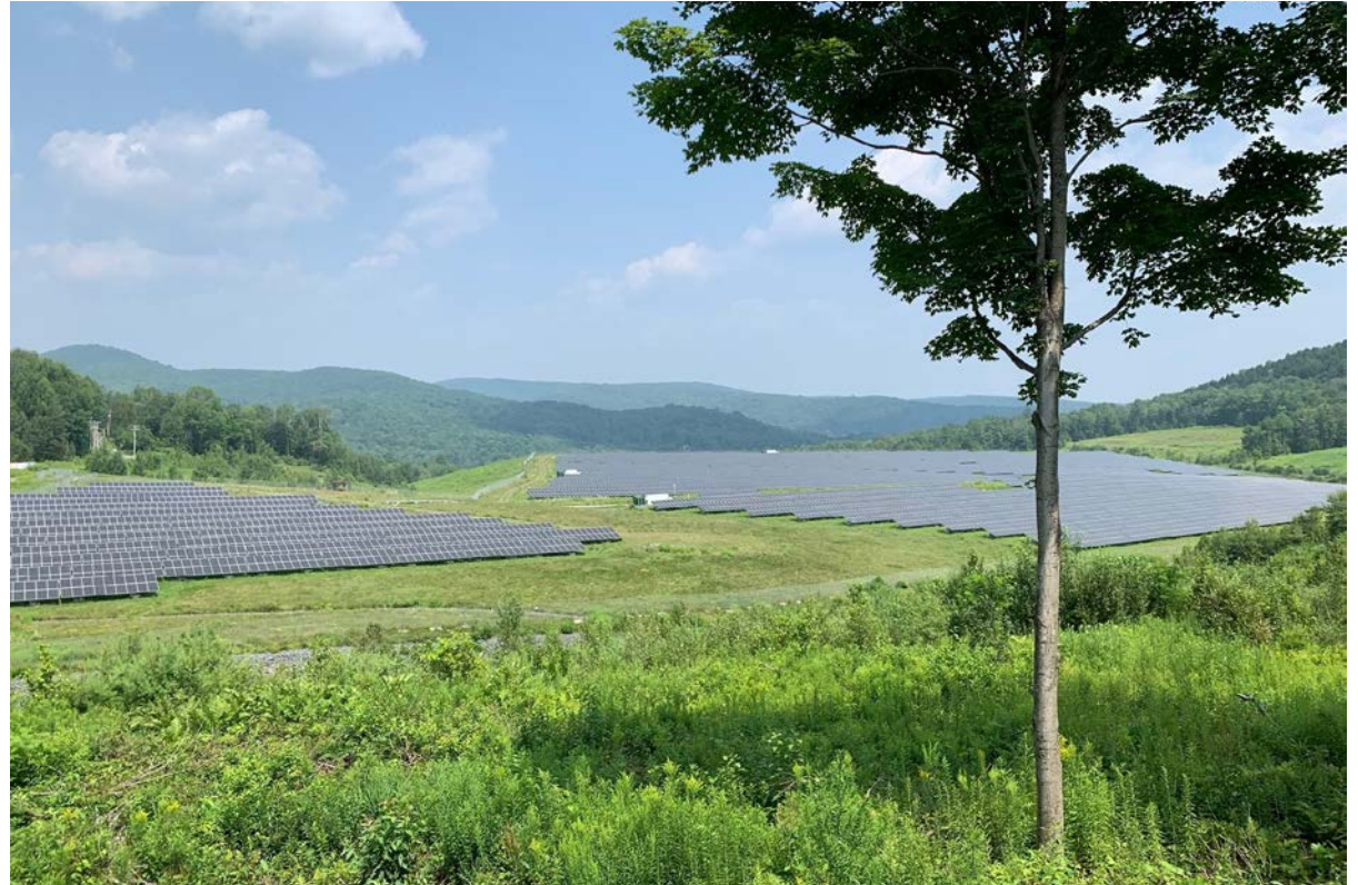
Solar Array at Elizabeth Mine Site | Source: Harry Falconer
