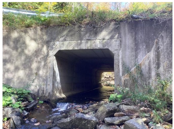
EXAMPLE OF BOX CULVERT Photo Credit: WRC
