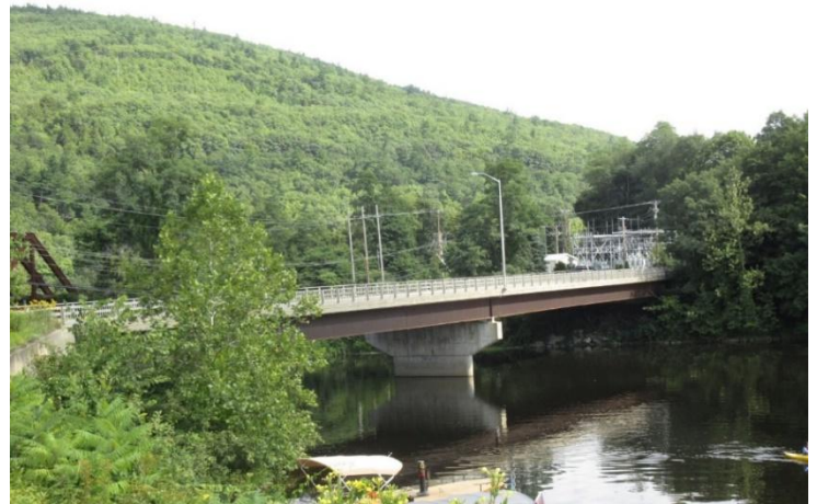
PUTNEY ROAD BRIDGE, BRATTLEBORO Photo Credit: WRC
