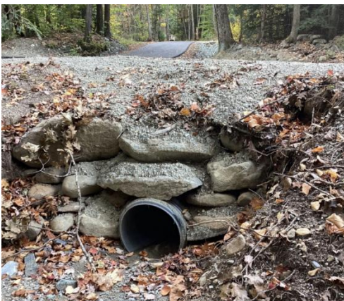
EXAMPLE OF ROAD CULVERT Photo Credit: WRC
