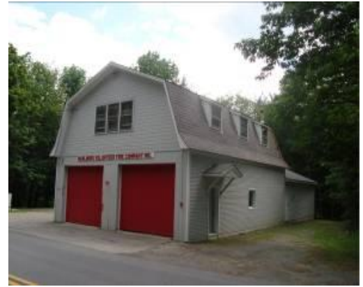
MARLBORO FIRE STATION
