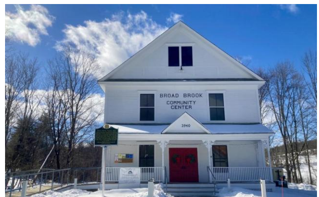
BROAD BROOK COMMUNITY CENTER, GUILFORD CENTER
